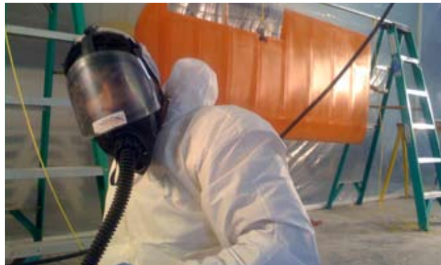
The HazMat painter. Steve tries to avoid permanent brain damage.
